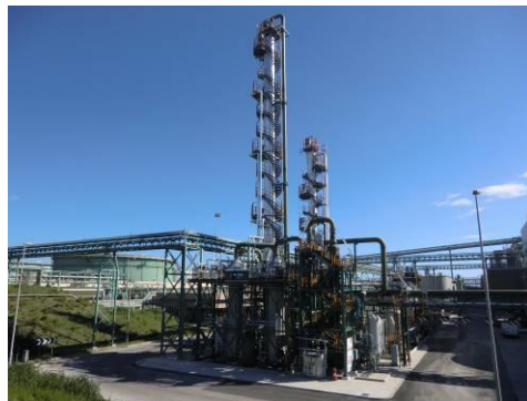
Figure 4: ENEL pilot plant in Brindisi (Italy) / Capacity: 2.25 TCO 2 captured/h
